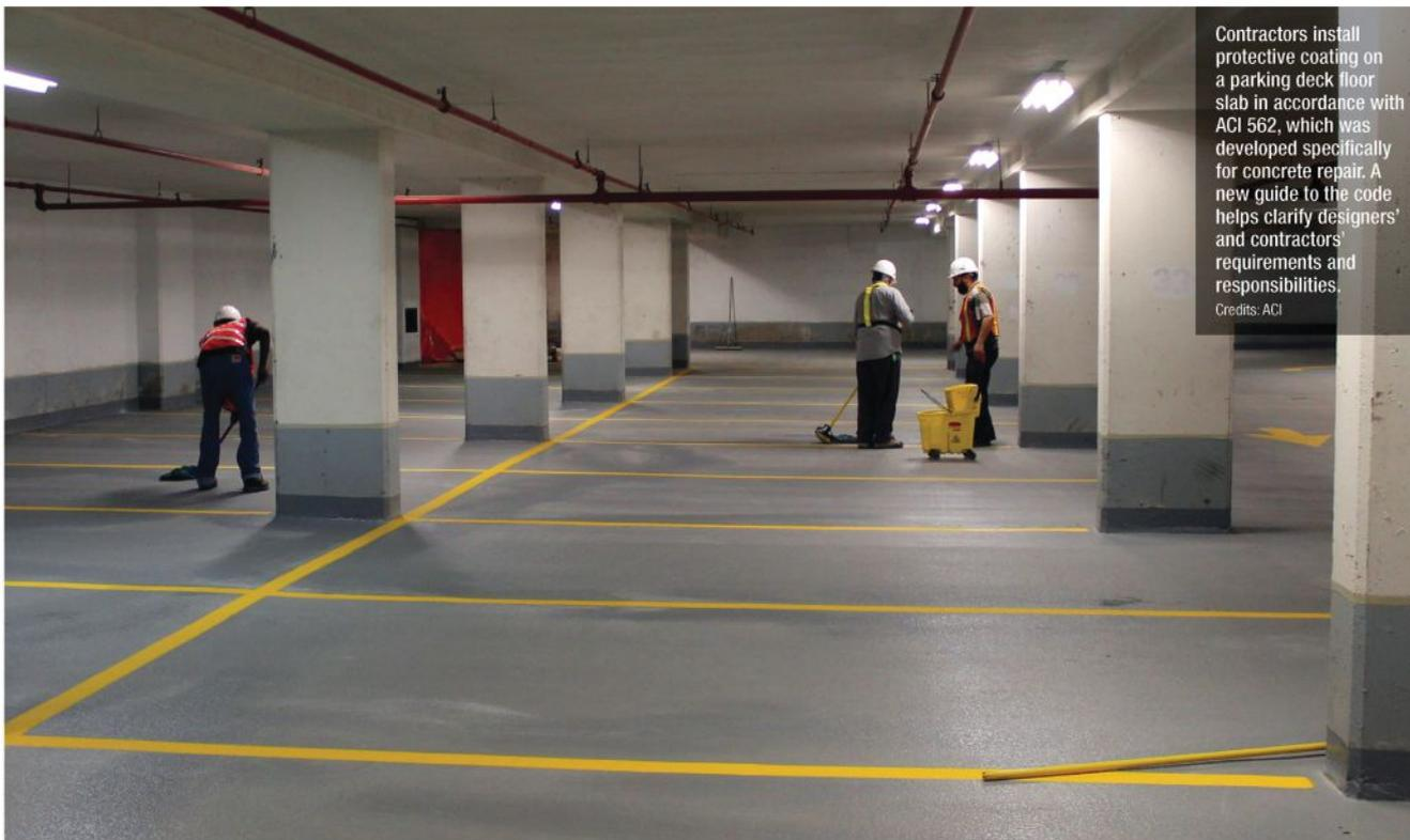
Contractors install protective coating on a parking deck floor slab in accordance with ACI 562, which was developed specifically for concrete repair. A new guide to the code helps clarify designers' and contractors' requirements and responsibilities.
